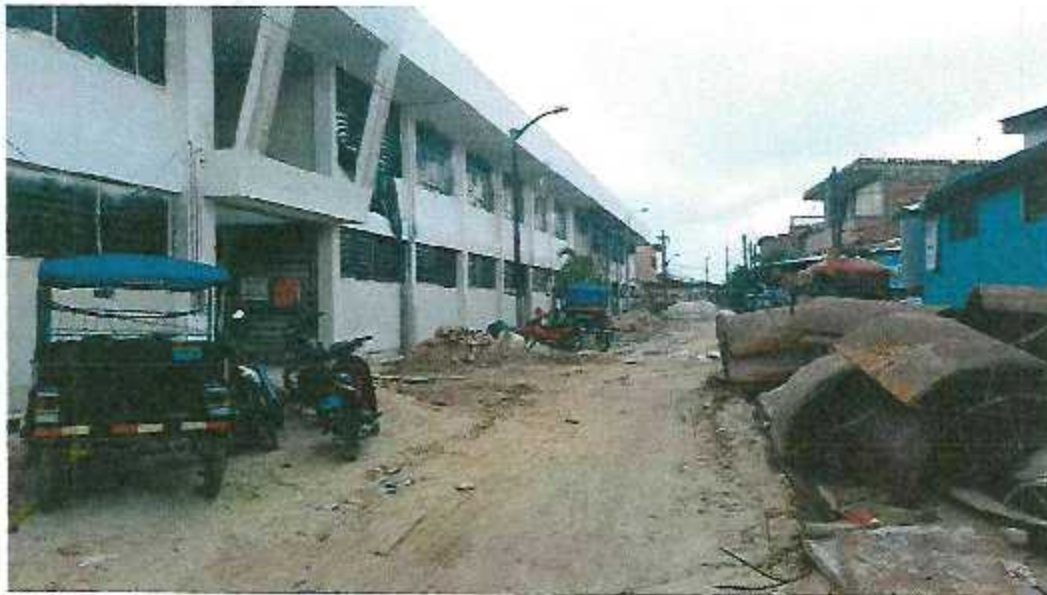
PINTURA LATEX EXTERIOR – FACHADA PRINCIPAL
